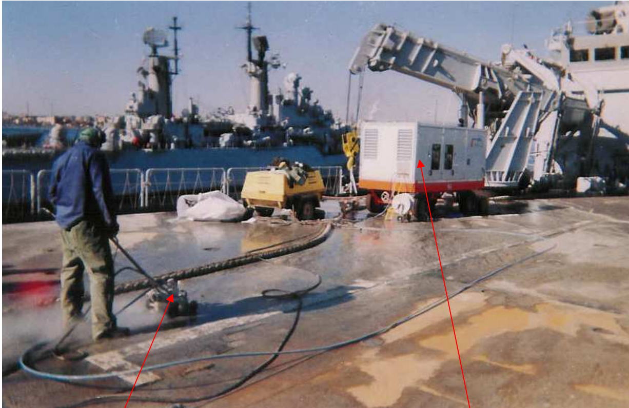
“Surface cleaner” in operation
