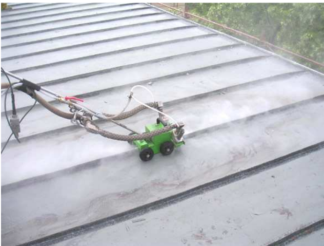
The KAMAT "Fold Cleaner FRG 2500" in operation at a construction site in Vienna, Austria
